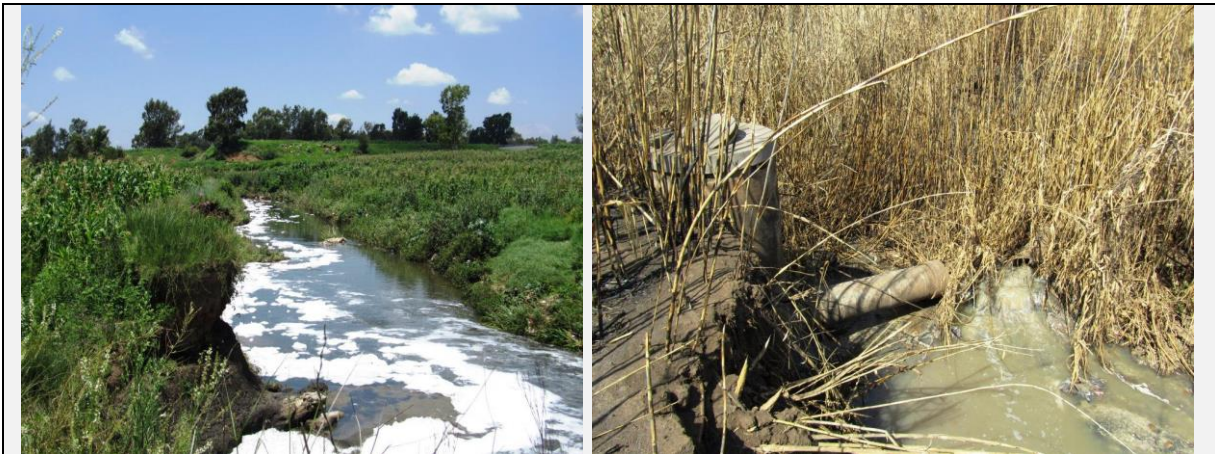
Figure 11: River condition a) Severe water quality conditions. b) Broken sewer line.
