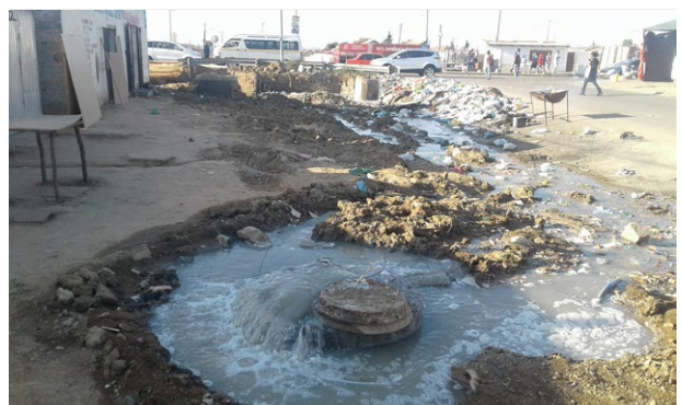
Blocked and overflowing sewerage main in Ivory Park running into the Kaalspruit.
