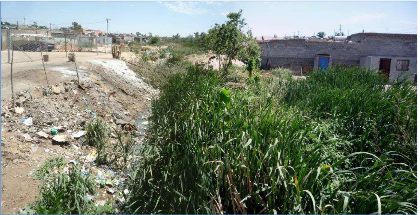
Figure 44, position 15: View north (upstream) from where Trout Street comes to the eastern edge of the steep, narrow drainage line of K2c Tributary, showing how roads and houses have constricted the watercourse from the east (right) and deliberate landfill from the west (left), yet bulrushes and some indigenous grasses and sedges survive within the stream bed.
