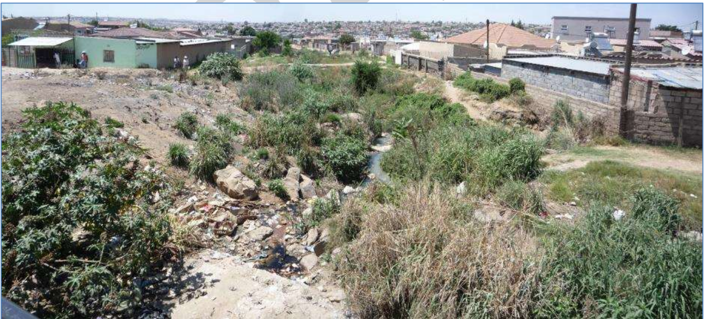
Figure 45, position 15: View south (downstream) from where Trout Street reaches the east (left) side of the drainage line of the K2c Tributary, constricted by landfill to the east and expanded housing to the west (right). Water still flows in the narrow bed and under an informal roadway, and bulrushes and other alien vegetation survive along its margins.
