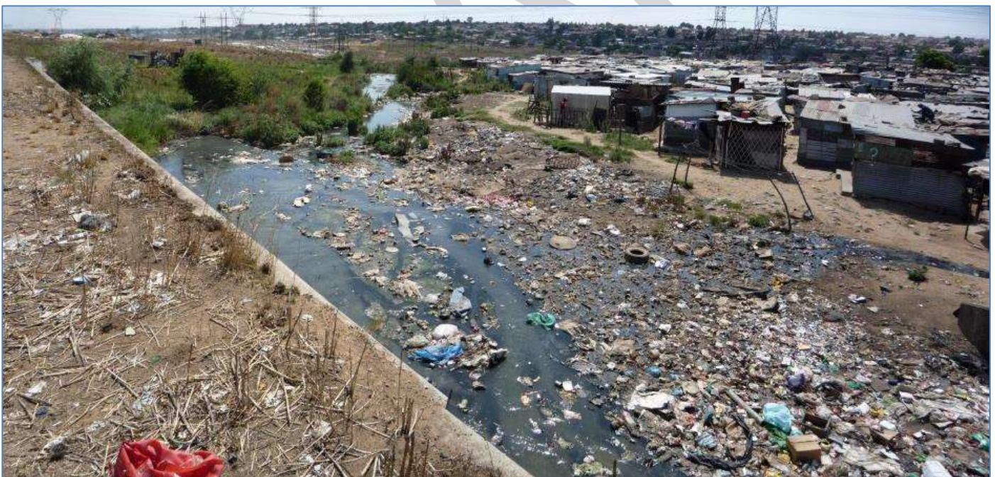
Figure 31, position 10: View east (downstream) towards where the K2 Tributary joins the northern section of the Kaalspruit mainstem in the valley floor below. Note the eroded river bed, total incursion of informal settlements and their waste on the south (right) bank, but the semi-natural though degraded vegetation on the north (left) bank.
