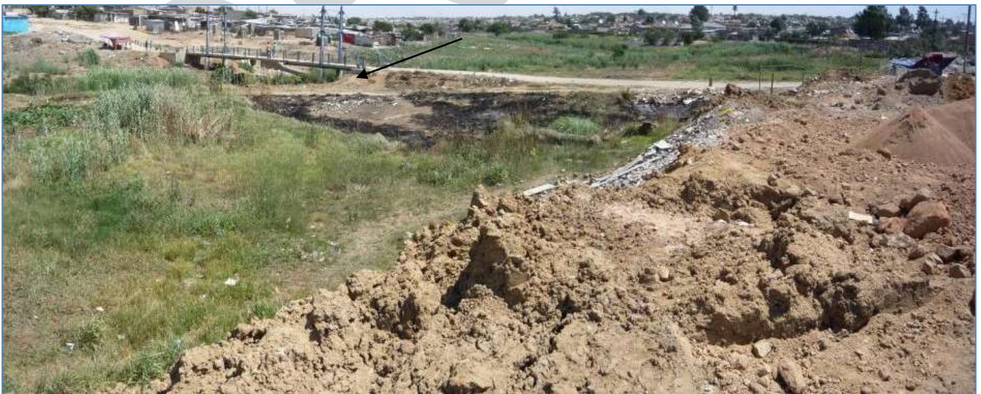
Figure 9, position: 1: View south (upstream) from an earth landfill into the west bank of the Kaalspruit River, west of its crossing of Freedom Drive, showing the reedy watercourse, grassy banks and low gradient upstream, with a pedestrian bridge and in the distance the southwestern Johannesburg-Ekurhuleni boundary. Note the constrictions on either side from the pedestrian walkway embankments.
