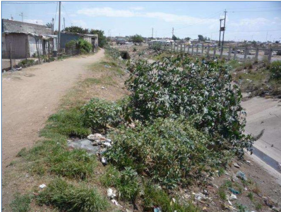
Figure 18, position 4: View south (upstream) along the concrete-lined canal to where the start of the open tributary emerges from a storm-water drain passing under 29 th September Street, but not as a distinct watercourse. Note the proximity of informal housing to the east (left) edge and tarred road to the east (right).
