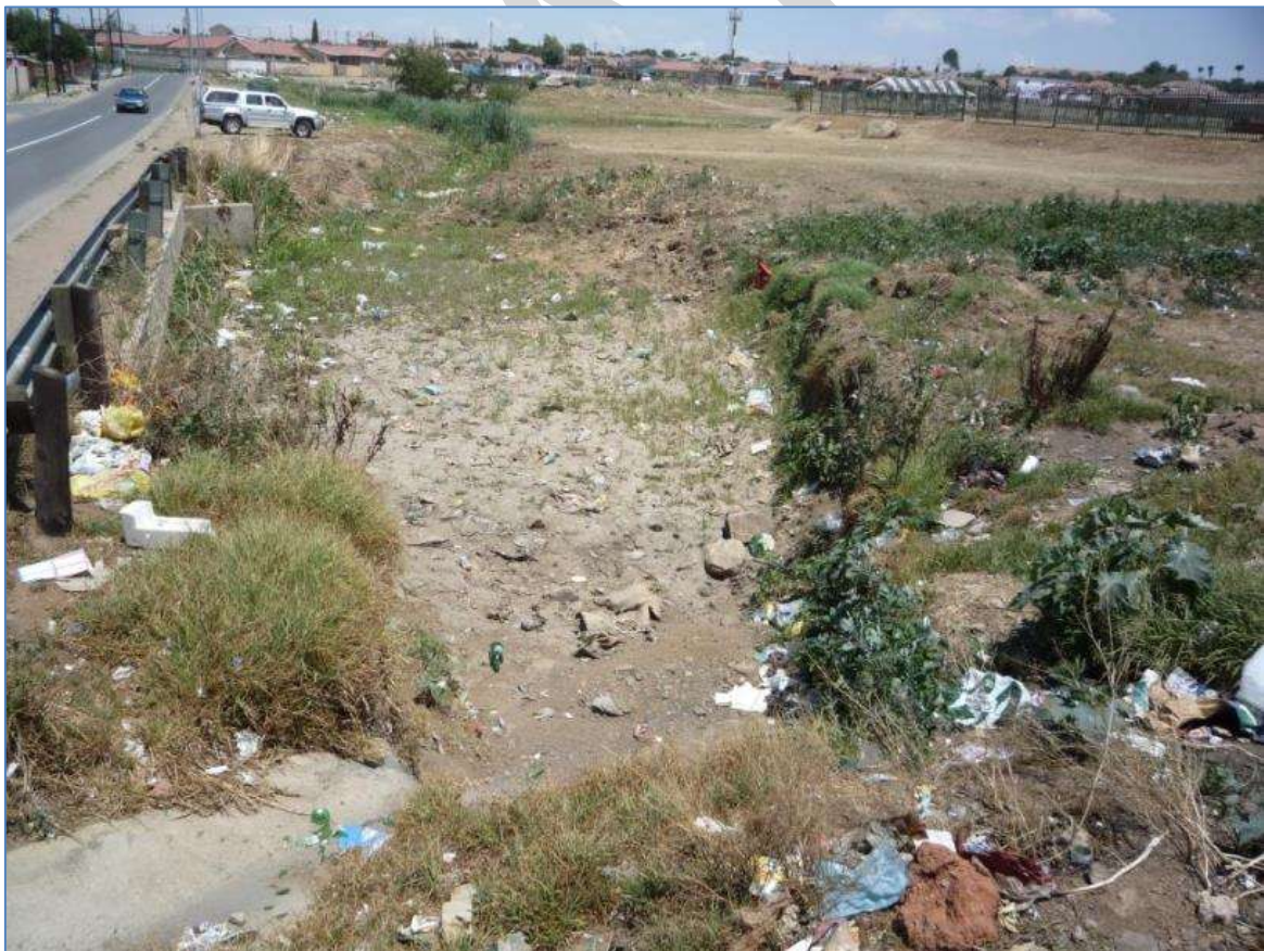
Figure 35, position 11: View along the west side of Camellia Street, showing where the drainage line of the K2a Tributary passes round the end of a landfill for a fenced recreation area and then re-enters its bed under the street. The narrow strip of green bulrushes that remains in the bed is fed by drainage of seepage/runoff from housing to the east (far side) of the tributary.
