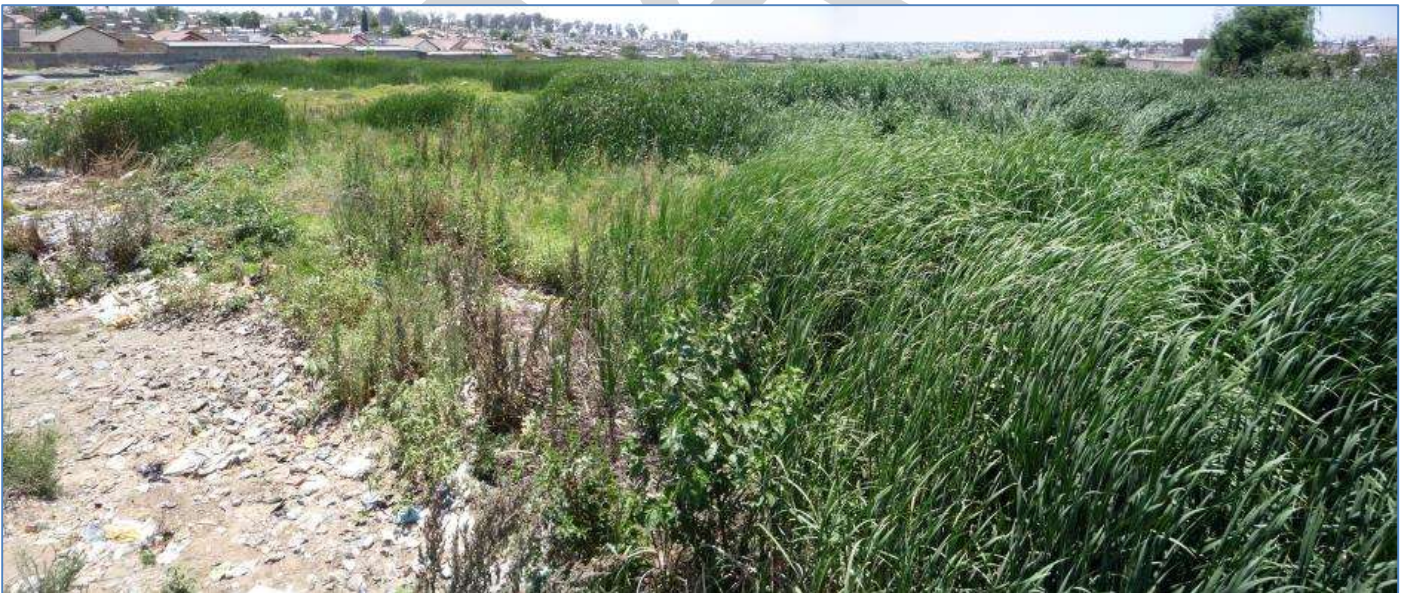
Figure 27, position 8: View east (downstream) along the K2 Tributary taken below its crossing under Archer Fish Street, showing where the drainage of runoff from the impermeable road surface has eroded and opened the outside of the bend, reducing the bulrush beds as their soils are washed away, with the streambed quality declining and giving way to reeds further downstream in the distance.
