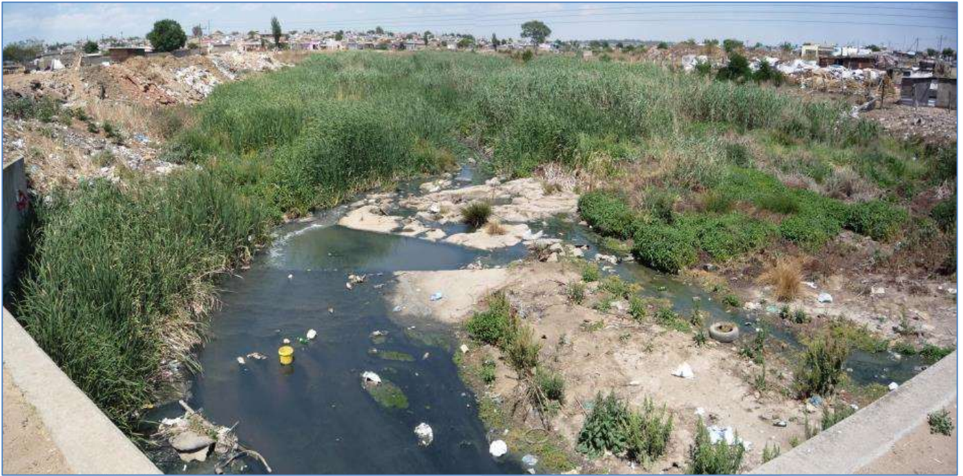
Figure 30, position 10: View west (upstream) where the lower reaches of the K2 Tributary pass under Republic (Main) Road. Note the encroachment of landfills and informal housing along the banks, the presence of some reed beds to stem water flow, and the obvious litter load.
