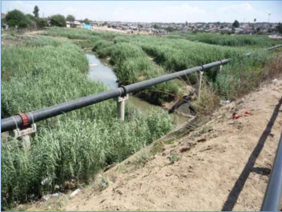
Figure 10, position 1: View south (upstream) from the crossing of the Kaalspruit River over Freedom Drive, showing the reed-filled watercourse, with a pipeline crossing in the foreground and the pedestrian crossing in the distance. Note the stream restricted to only one of several channels due to late rains. Note the damming effect of the road embankment (cf. Fig. 11).
