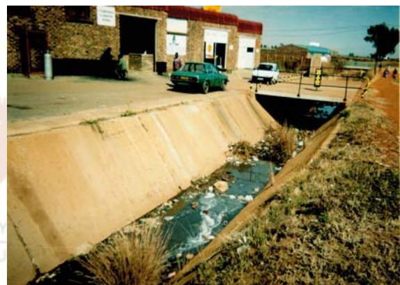
Figure 6: Clayville concrete channel
